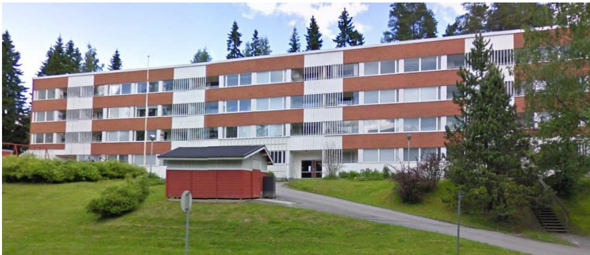
Figure 10 - The apartment building chosen for the demonstration represents a typical example of Finnish housing from 1970s.
