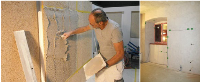
Application and monitoring of the Lime Mortar
