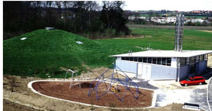
Fig. 04: 1st Generation - Friedrichshafen (1996); (source: solites)
