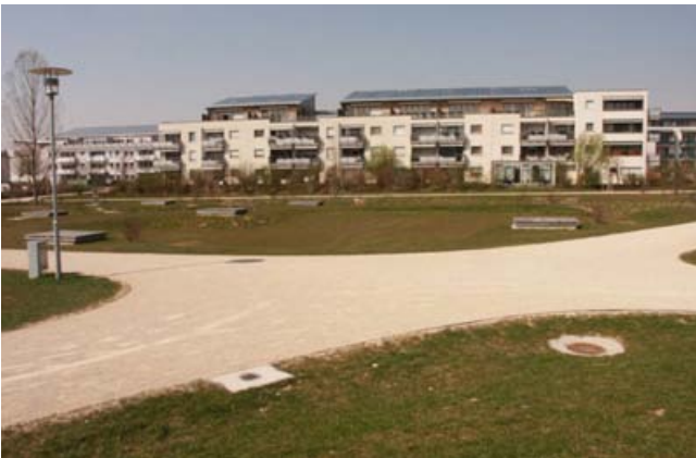
Fig. 32: Example of the open space design of borehole thermal energy store (source: solites)
