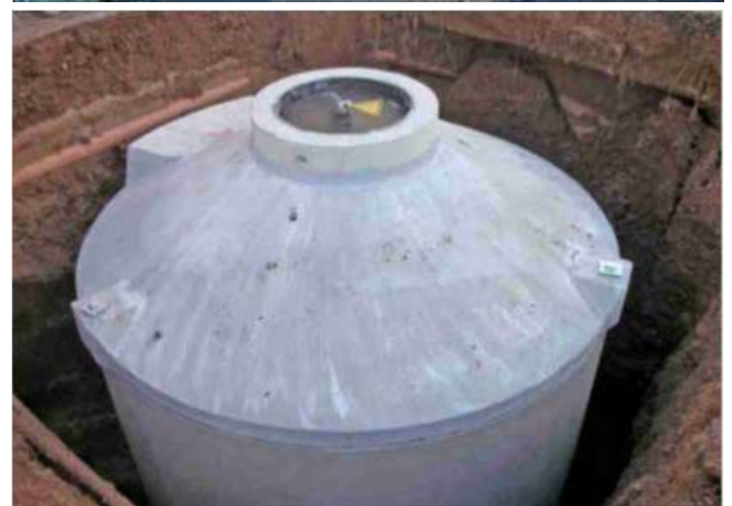
Fig. 45 and 46: Thermosol store of company Mall (source: Mall Umweltsysteme)
