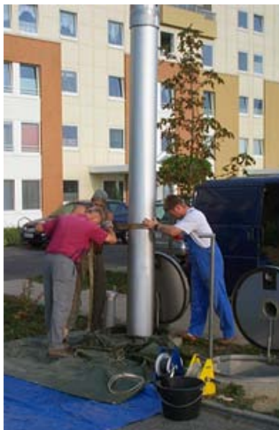
Fig. 34: Installation of the well pipe (source: solites)
