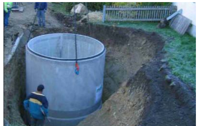
Fig. 43: Glass fiber reinforced plastic (GRP) tanks of company Haase (source: Haase GFK-Technik GmbH)
