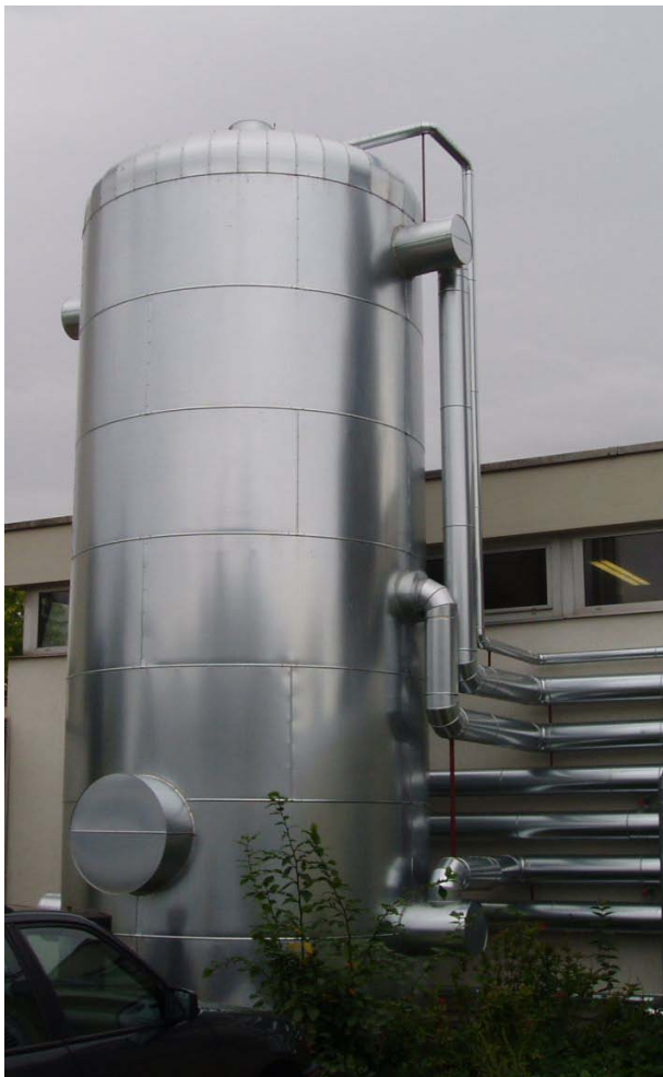
Fig. 52: Buffer storage, baths Koll (source: solites)
