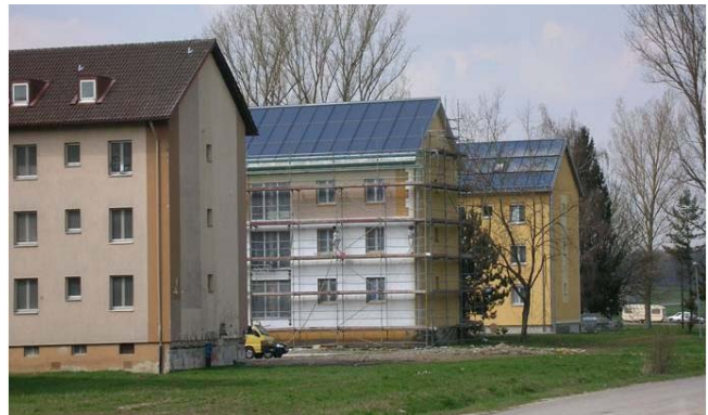
Fig. 55: Realization of a comprehensive energy concept applied on former army buildings in the STES pilot system in Crailsheim, Germany: with the realization of a solar assisted district heating net with STES the existing buildings were energetically retrofitted. (source: Solites)
