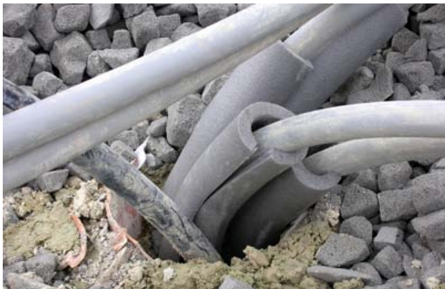
Fig. 26: Insulation of geothermal probe pipes (source: solites)
