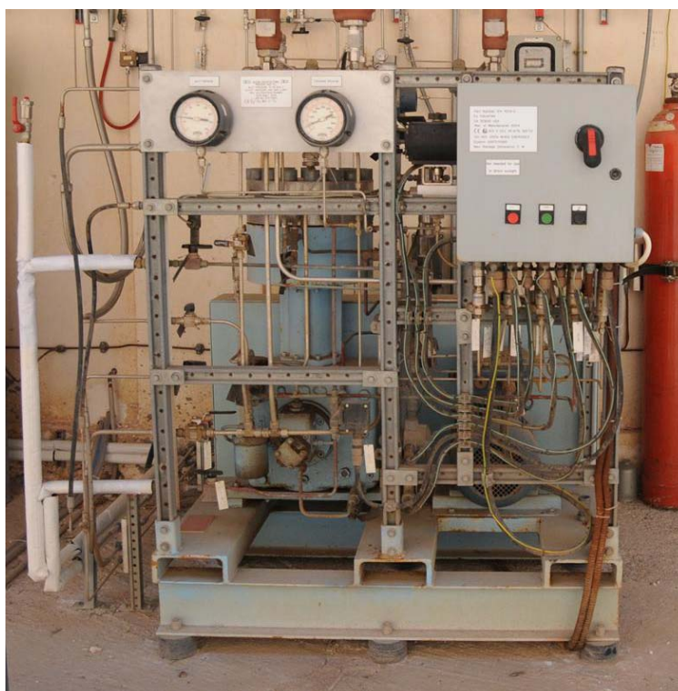
Figure 4. H 2 compressor.
