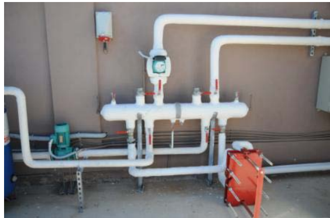
Figures 7 (left) and 8 (right). HRS “puffer” tank and plate heat exchanger connected to HVAC unit respectively.
