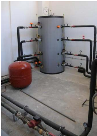
Figures 7 (left) and 8 (right). HRS “puffer” tank and plate heat exchanger connected to HVAC unit respectively.
