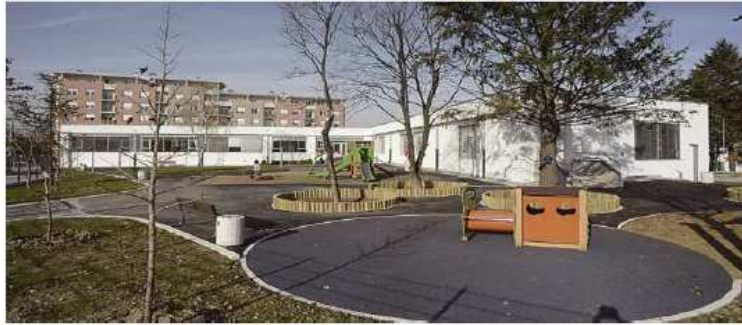
Figure 13. Kindergarten/Children facility "Mala Sirena"
