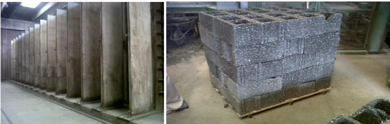
Curing rooms and stocking of the blocks.
