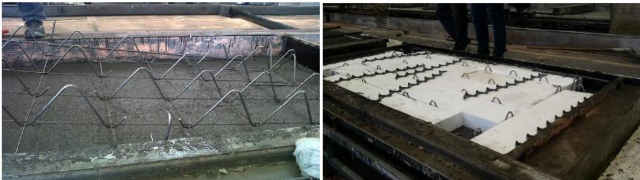
Metallic reinforcement and positioning of EPS100.
