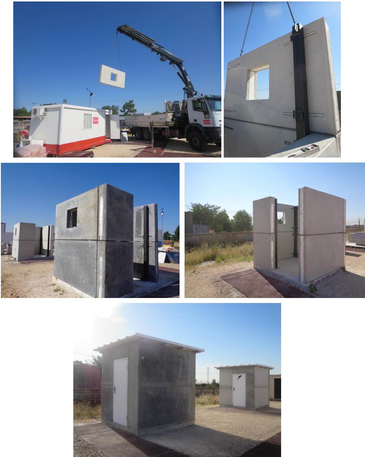
Figure 9: Mockups built with panels: SUS-CON panels (front) and traditional panels (back).
